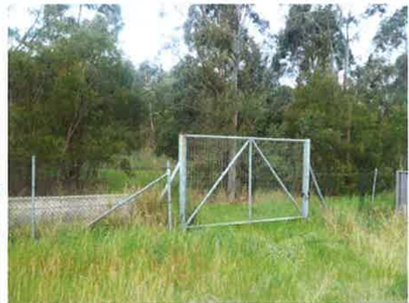
Figure 3: Site showing access gate no longer required by the RTA for access to the land to the east (used for construction of the bypass only)
