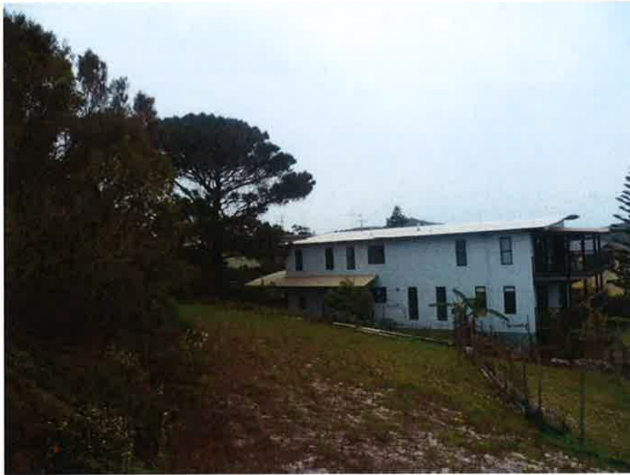
Figure 4: Site showing Squire Street frontage looking ENE.
